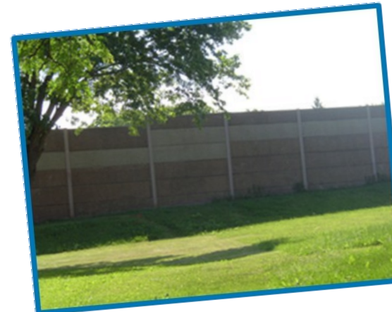
View of Noise barrier from the residential side.
